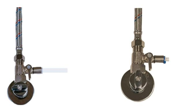
We will leave the supply valve of the osmosis equipment in the closed position and proceed to open the supply square valve of the sink tap, so we can verify that there are no leaks.
