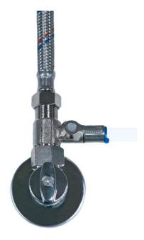
We will open the service tap of the equipment, we will leave it open for 5 minutes. If it is observed that the water that comes out in these first minutes has a dark color, it is completely normal, it is the rinsing of the filters.
